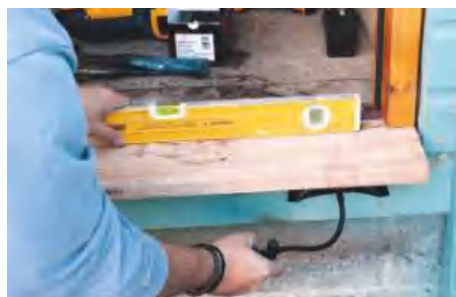
▲ It's equally simple to lift the frame as a unit or to adjust one side for level
